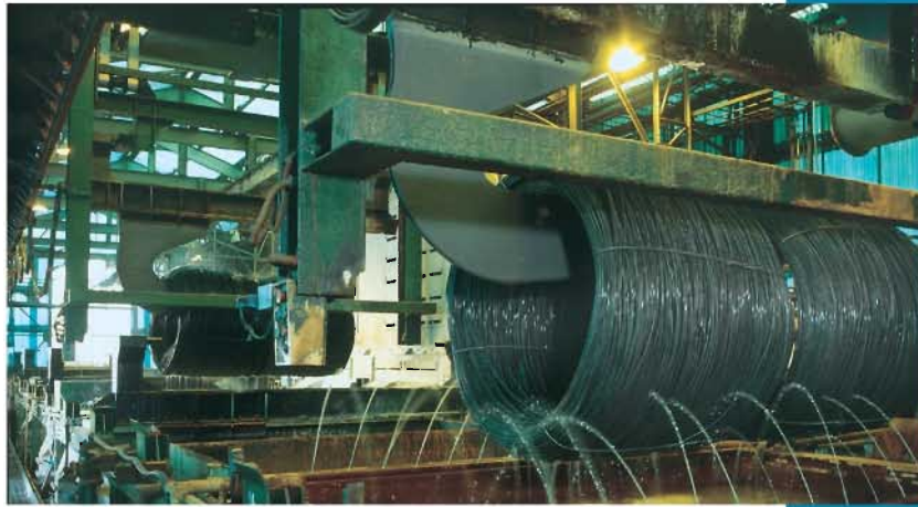
PLC operated modern pickling plant
