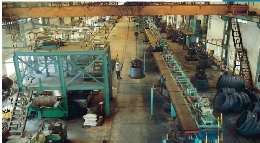
PLC operated modern Patenting-cum-galvanising line
